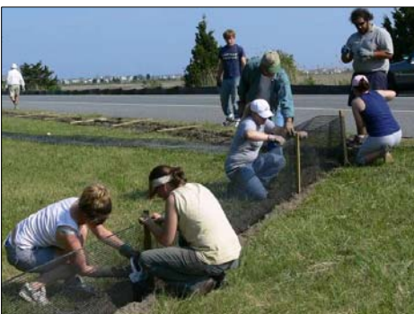
Wetlands Institute volunteers installing barrier fencing to prevent terrapins from crossing roadways.
