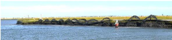
Figure 3 - Trialing techniques to build elevation and marsh edge protection with cohesive sediments at Sturgeon Island.
