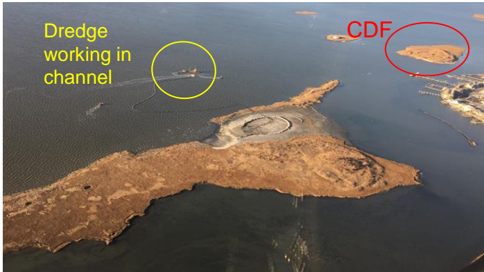
Mordecai Island Restoration Beach Haven NJ (2015 and 2017)
